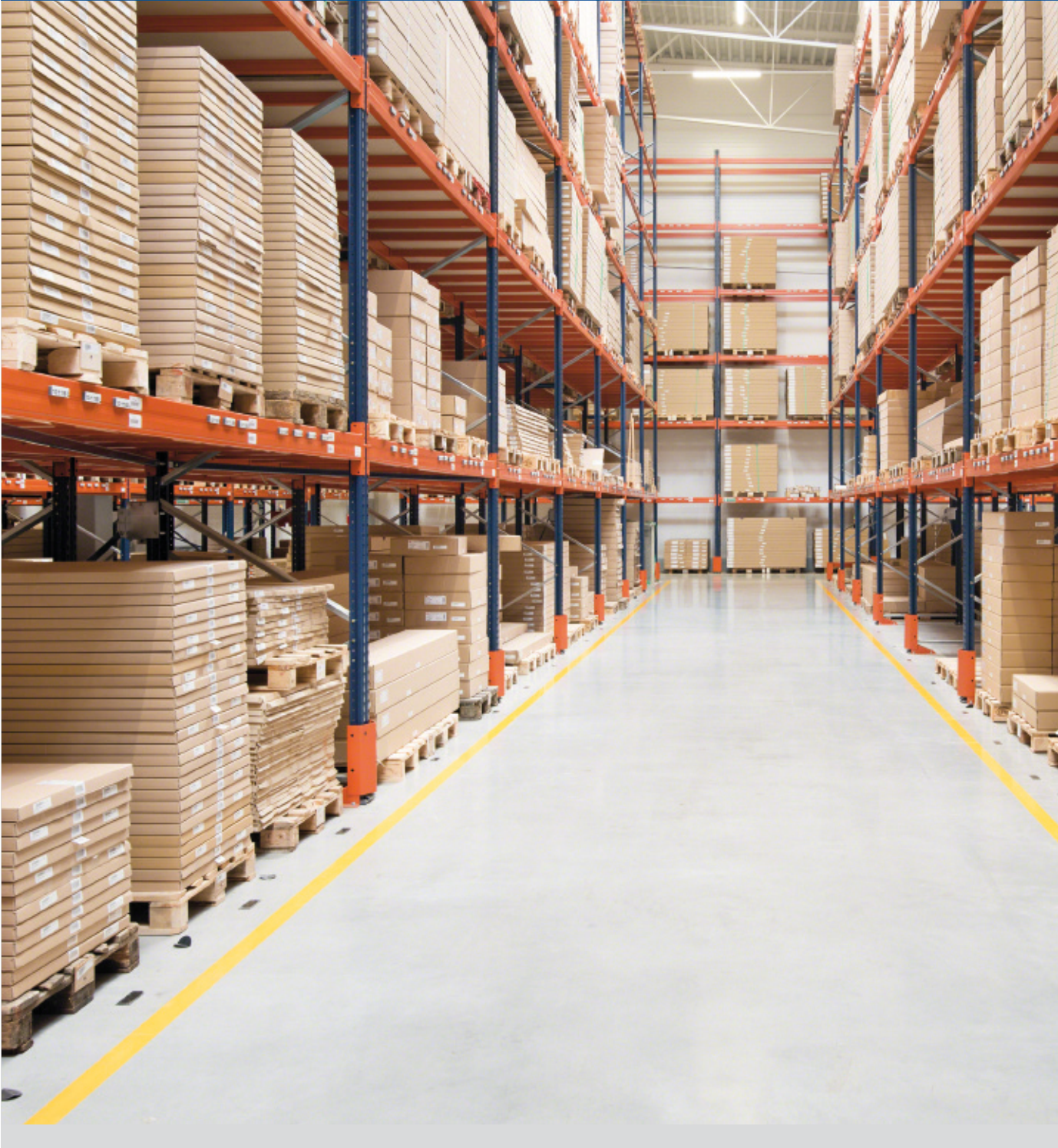
Mecalux has installed pallet racking in the new warehouse Dolmar owns and operates in Kepno (Poland). In addition to providing direct access to merchandise, which streamlines storage tasks, this system houses 6,445 large-sized pallets.
