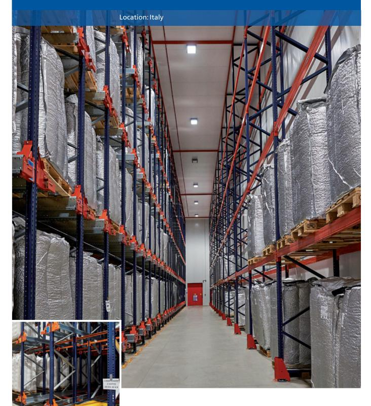
The new 3PL warehouse of Katoen Natie in Italy comprises pallet racks and the semi-automatic Pallet Shuttle system of Mecalux. These solutions max out space usage by providing a 7,765-pallet storage capacity. Racks are reinforced to protect workers and the goods from potential seismic tremors.
