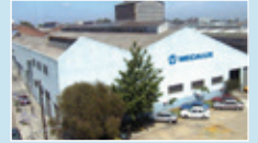
Plant in Buenos Aires, Argentina
