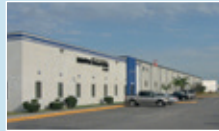
Plant in Matamoros, Mexico
