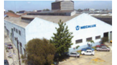
Plant in Buenos Aires, Argentina
