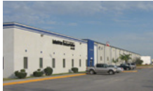
Plant in Matamoros, Mexico
