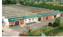
Plant in Palencia, Spain
