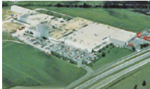
Plant in Pontiac, US
