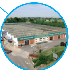
Palencia plant (SPAIN) 23,500 m 2
