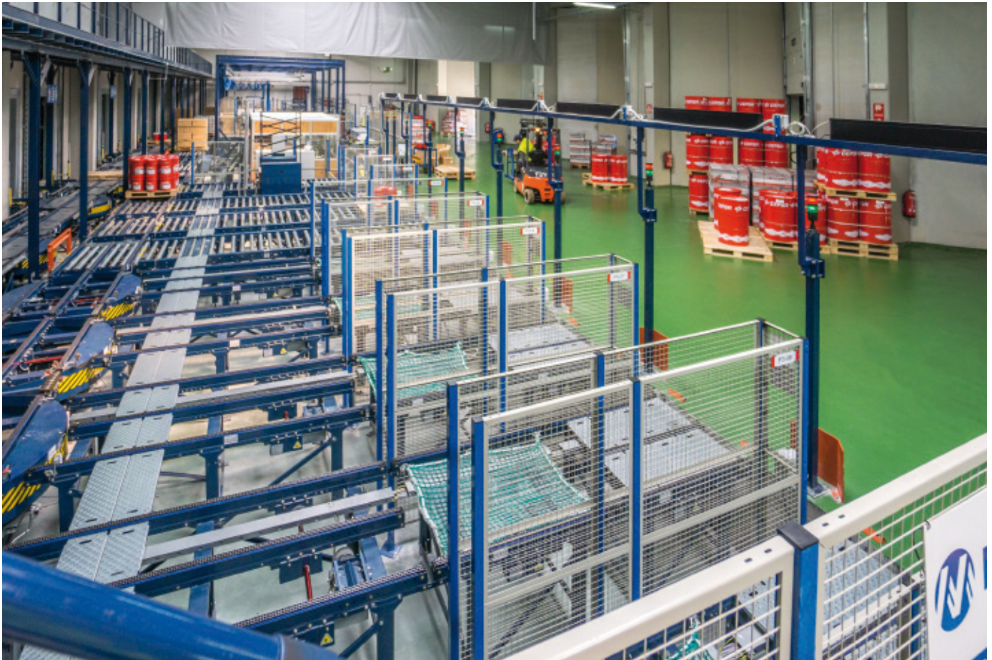
View of the dispatch area
