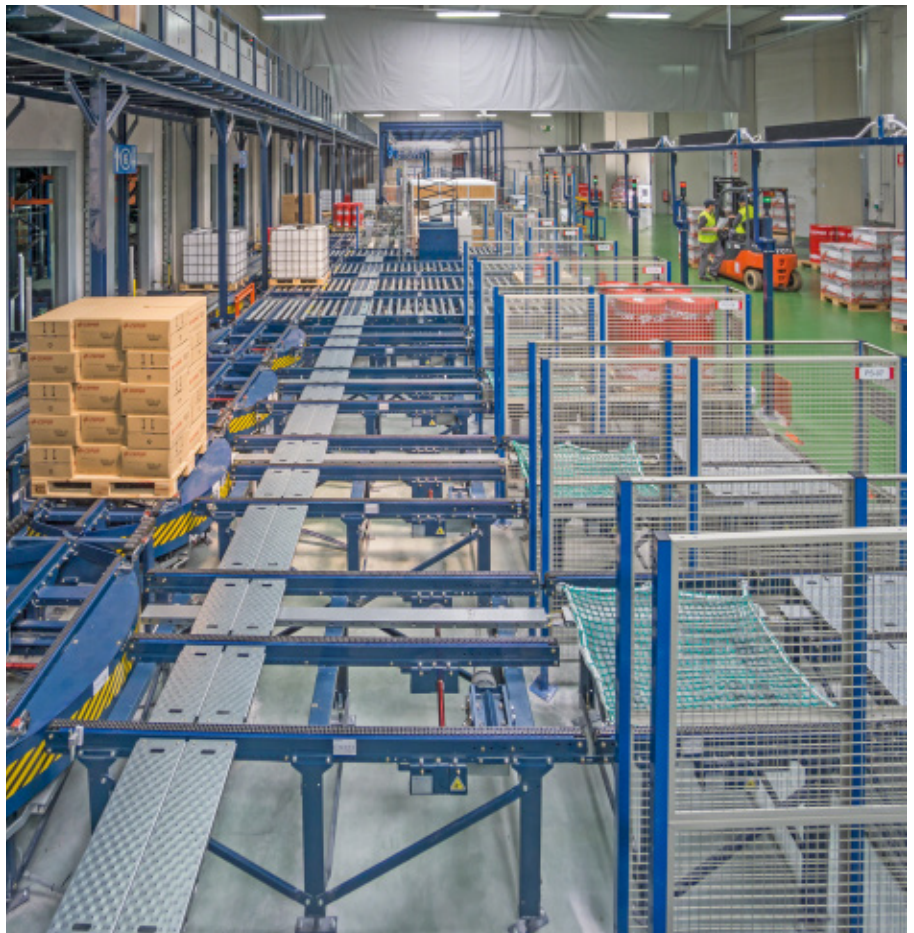
View of the main dispatch conveyor
