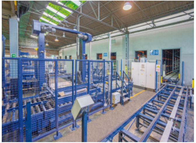
Production conveyors and warehouse access
