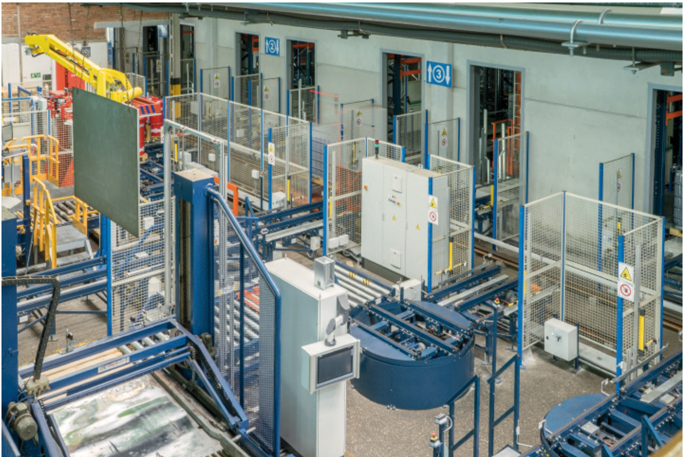
Conveyor and entrance to the production warehouse
